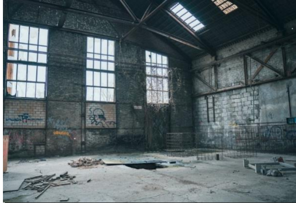
Figure 5. Abandoned warehouse. Koln, Germany. Timo Scheiler, 2023.
