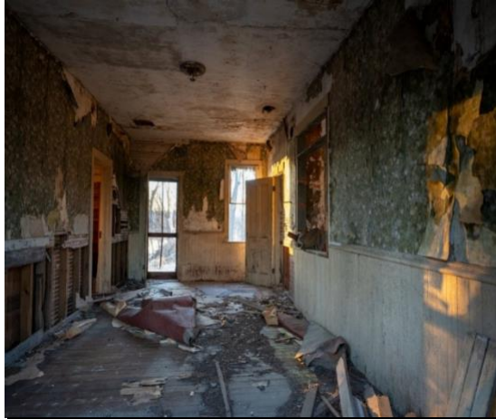
Figure 1. Abandoned interior. West Newton, MN. Tom Fisk, 2021.
